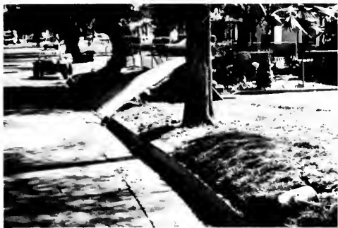
Photo 12. Adelphia Street in fault zone, San Fernando, view south-east. Spectacular left-lateral displacement of curbing accompanied by compression of driveway.
